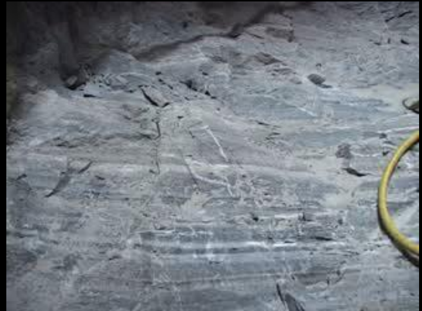
Harlem River Tunnel - 2009
