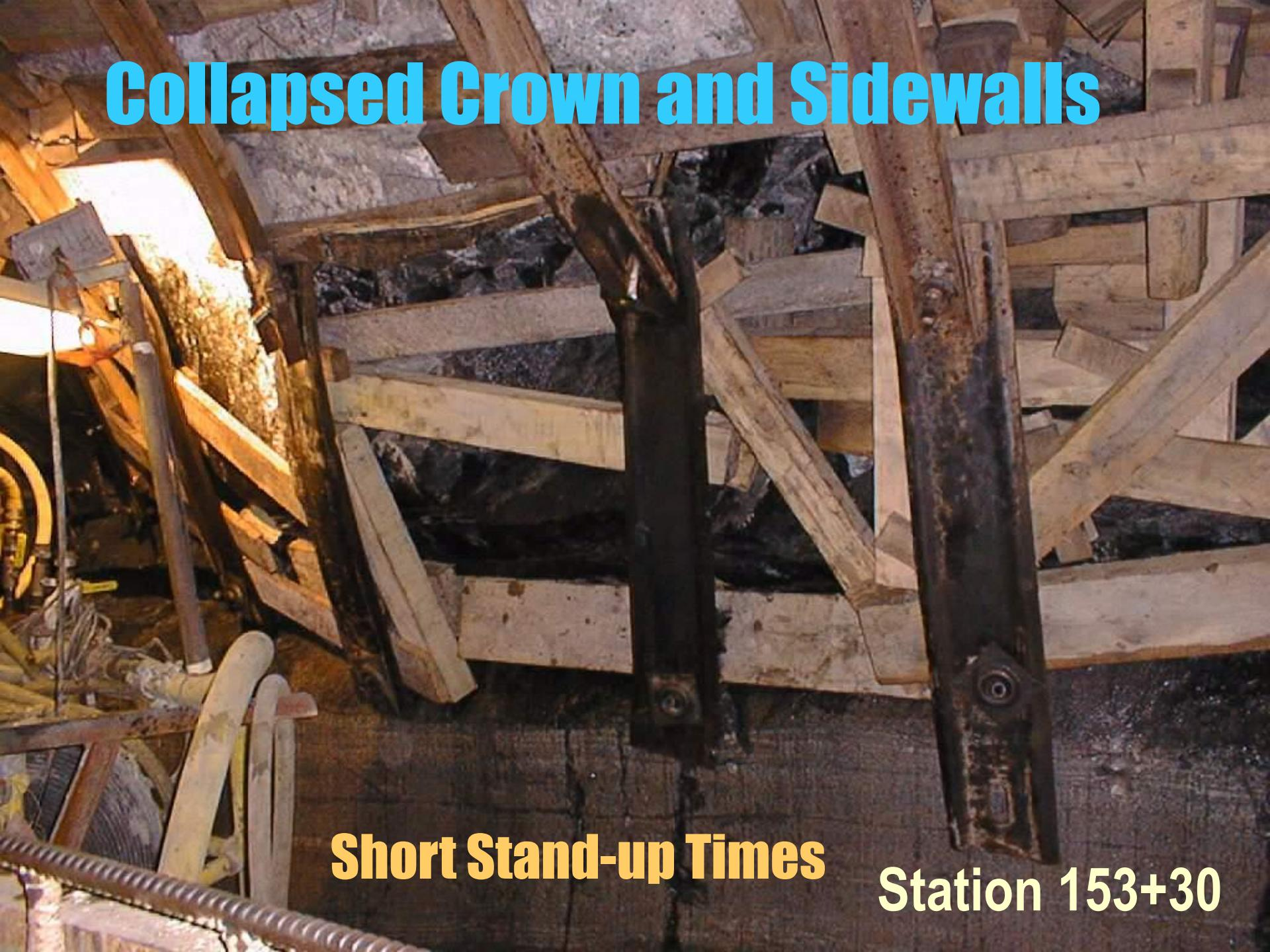
A photograph of a collapsed tunnel or excavation site. The image shows a dark, cramped space with wooden timbering and metal support beams. A large amount of dark, crumbly debris is visible, indicating a collapse. The lighting is dim, with some brighter areas from artificial lights.
