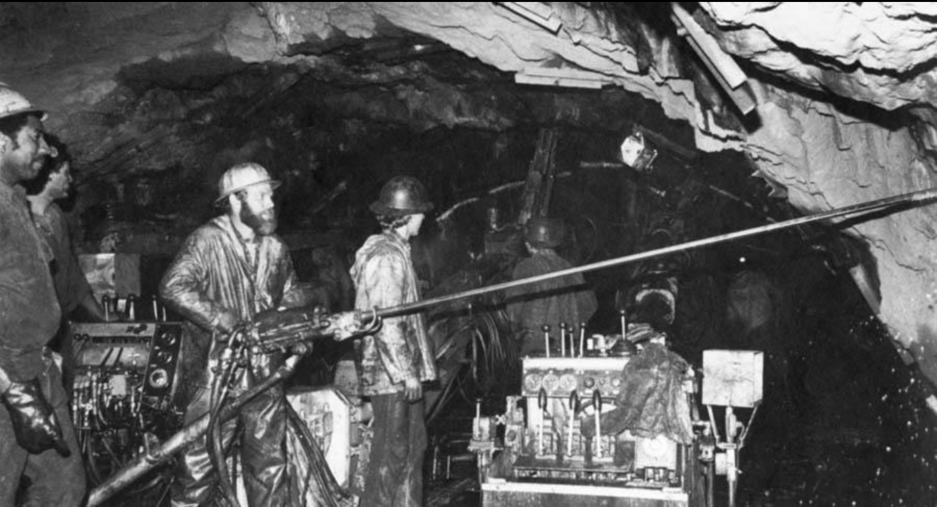
City Tunnel #3, Stage 1 – Drill and Blast Technology
