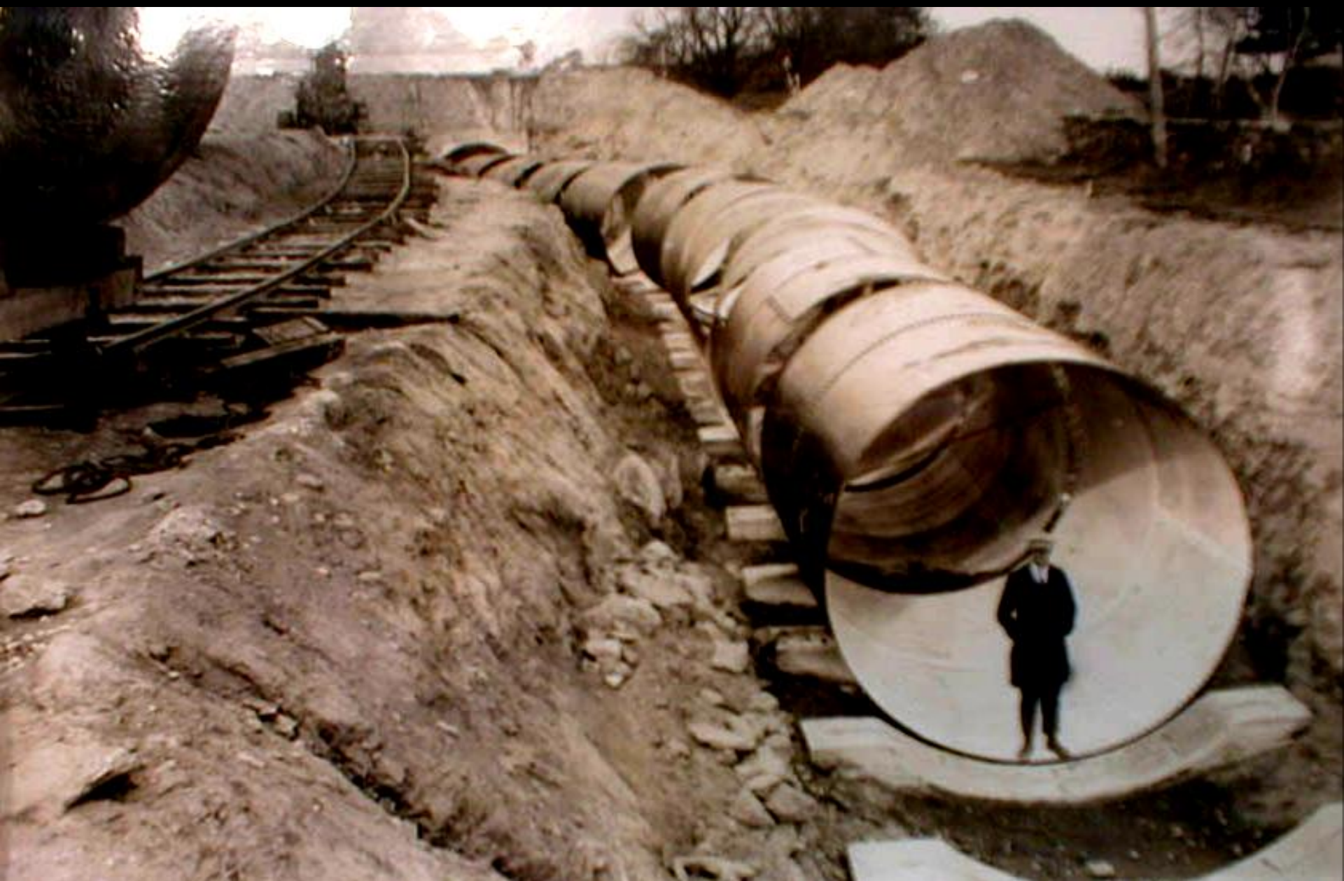
Cut and Cover Tunnel, NYC Aqueduct
