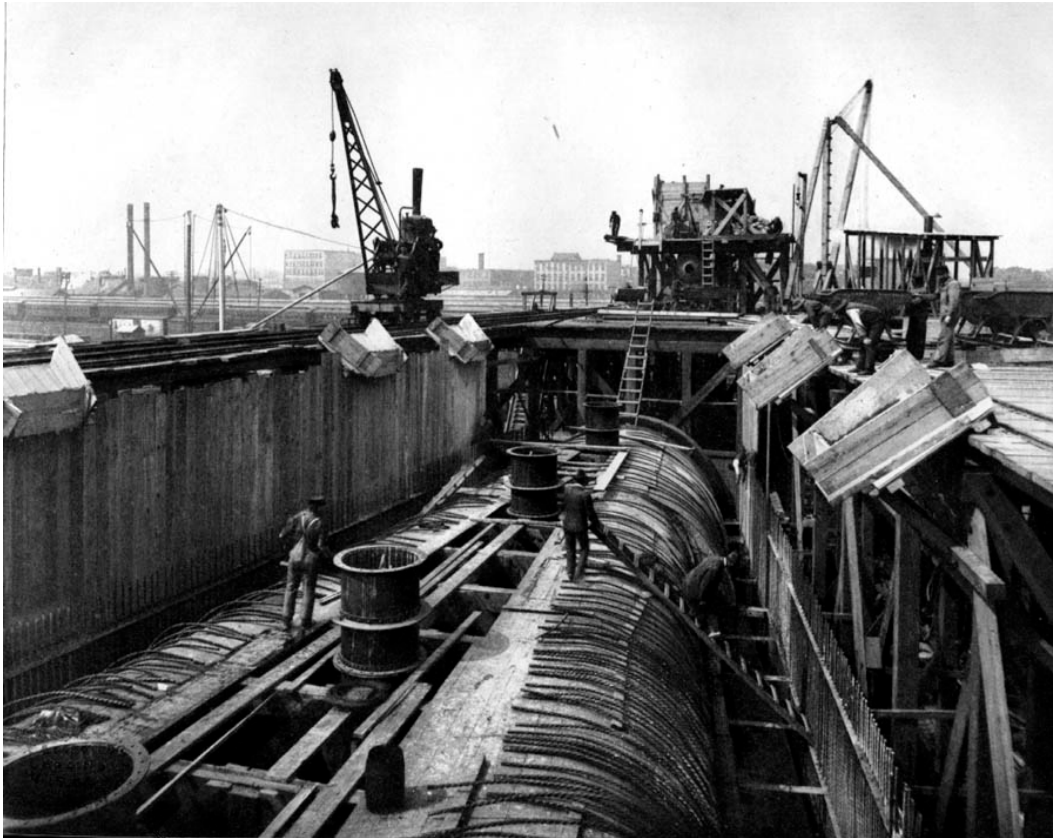
Figure 5 – Sunken tube technology dates back to the 1909 construction of the Hudson River Railroad Tunnels (now PATH) connecting lower Manhattan with New Jersey. (Archival image.)
