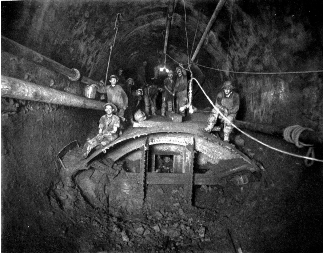
Figure 8 – Mechanical mole (TBM) of 1909 vintage, used to excavate the Hudson River Railroad Tunnels (now PATH) connecting lower Manhattan with New Jersey. (Archival image.)
