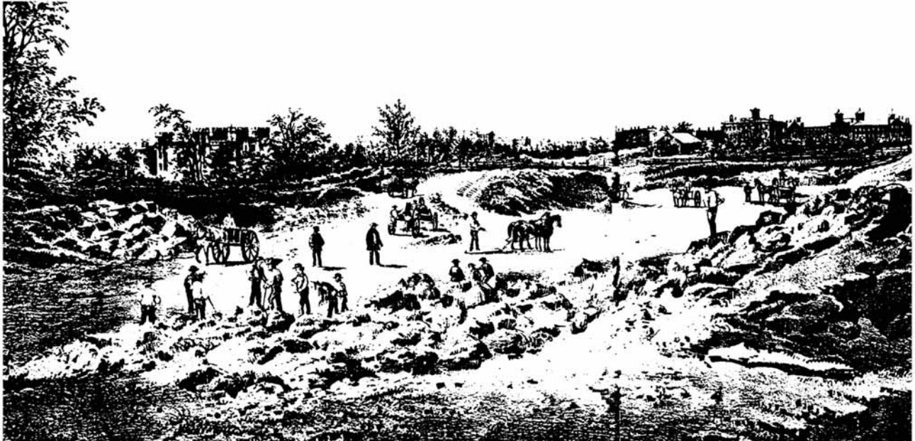
Figure 1 - View toward the south in 1858 of men with pick and shovel with horse carts clearing away the Pleistocene boulders during an early phase of construction of the Olmstead and Vaux "Greensward Plan" for Central Park in New York City. From left to right, the standing buildings include the Arsenal at 65 th Street and Fifth Avenue, the Catholic Orphan Asylum for Boys between 51 st and 52 nd Streets, and St. Luke's Hospital between 54 th and 55 th Streets. (Unidentified drawing from Laredo and Reed, 1979, p. vi-vii.)
