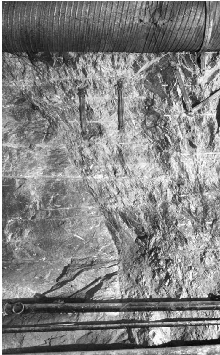
Figure 33 - Photograph of the 125 th Street fault as exposed in the subsurface of Manhattan in the water tunnel built roughly 250 m beneath Amsterdam Avenue. Note the sharp demarcation of the fault. The photo, by Carl Ambrose of the NYC DEP, covers roughly 7 m in vertical dimension and shows the presence of ventilation, compressed air, and electrical conduits along the top and bottom and bolted rock straps to hold up the fractured bedrock. (NYC Bureau of Water Supply photo.)
