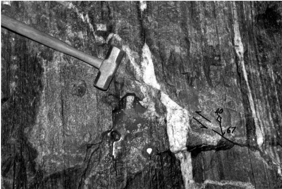
Figure 32 - Photograph of a left-lateral strike-slip fault exposed in the New York City water tunnel beneath the east channel of the East River between Roosevelt Island and western Queens. The fault is oriented N20°W, 67°NE and shows 7 cm of left-lateral offset in a quartz segregation within the Fordham Gneiss Formation.
