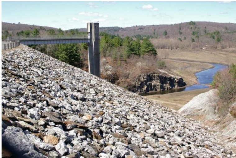
Figure 24. View of the N side of Thomaston Dam. The surface is armored with large boulders of white pegmatite and gray schist. (H. Moritz photo.)
