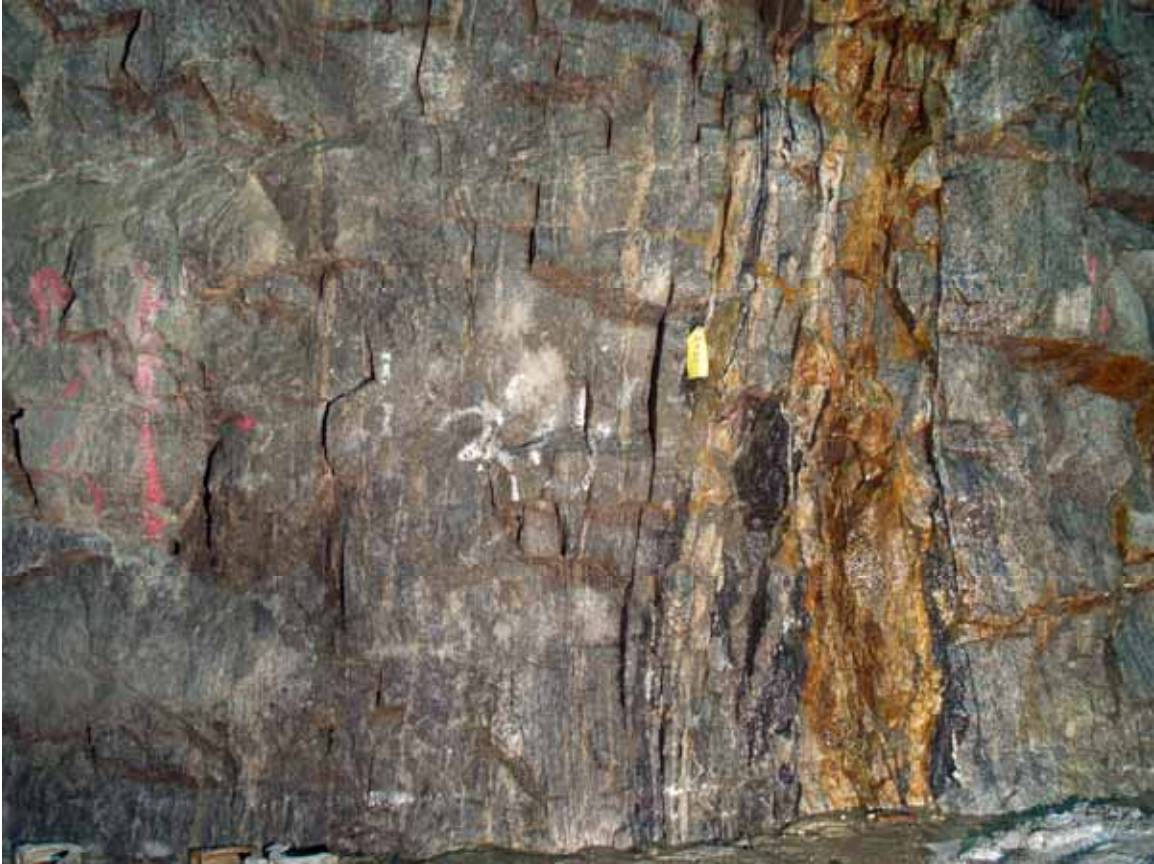
Figure 7 - Typical Yonkers Gneiss (Zy). Station 5+50, north wall raw water tunnel, Croton Water Treatment Plant, Bronx, New York. (Digital image by C. Merguerian).
