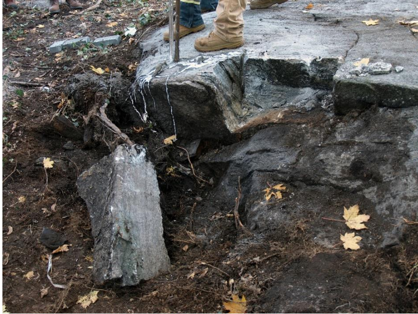
Figure 22 – Workers prying loose bedrock pieces easily with pry bars after pulse #2. After removal from the pulse zone, the broken pieces (Figure 23) together accounted for roughly 1.8 cubic yards of rock removed after the second pulse. (Dukelabs image taken 17Nov21.)
