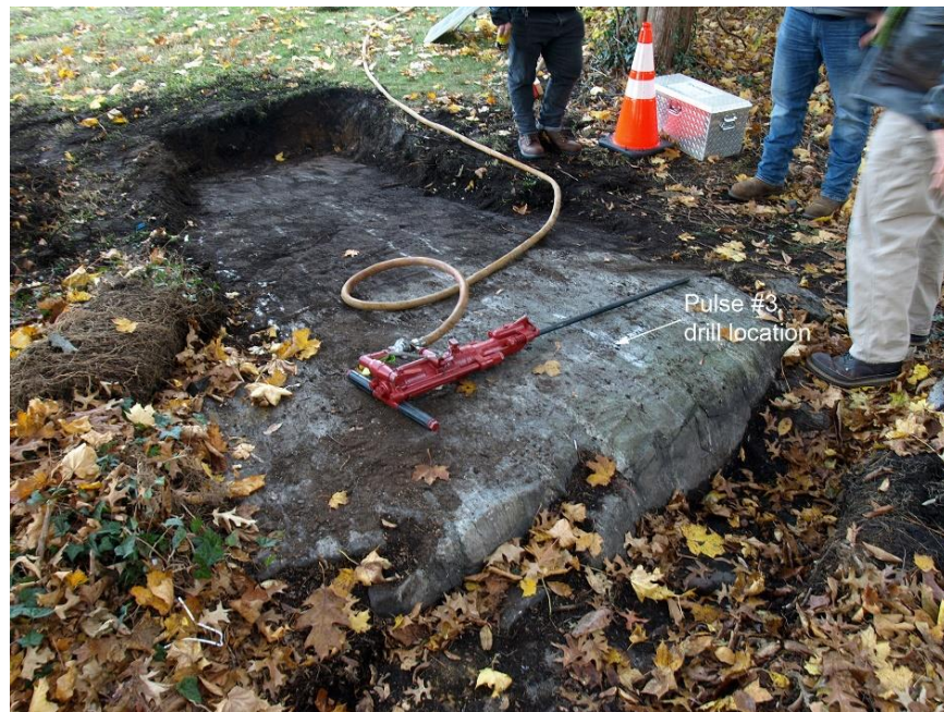
Figure 24 – View of partially open face of outcrop at Site #3B showing the location of the probe hole to be drilled by crew. (Dukelabs image taken 17Nov21.)
