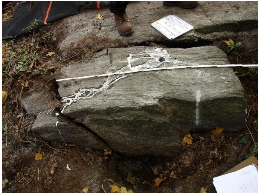
Figure 19A - View of dislodged 0.58 yard 3 block of Hartland gneiss that moved up and out from exposure the result of pulse #1. Failure took place along surrounding joints which were weathered, filled with soil and roots and seem to have absorbed and localized pulse energy. The shape of the block is controlled by the geological surfaces S 1 , J 1 , J 2 , J 3 and J 4 as shown below in the annotated view of the same block. The block was moved easily with a backhoe and later broken into smaller pieces by the backhoe bucket. (Dukelabs image taken 17Nov21.)
