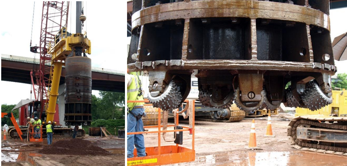
Figure 2 – Westward view of Shaft #23 construction rig near Pier 3 of job site in New Jersey (L) and close-up view of the cutterhead and cutters (R) designed for sedimentary rocks. (Dukelabs digital images taken 14 June 2013.)
