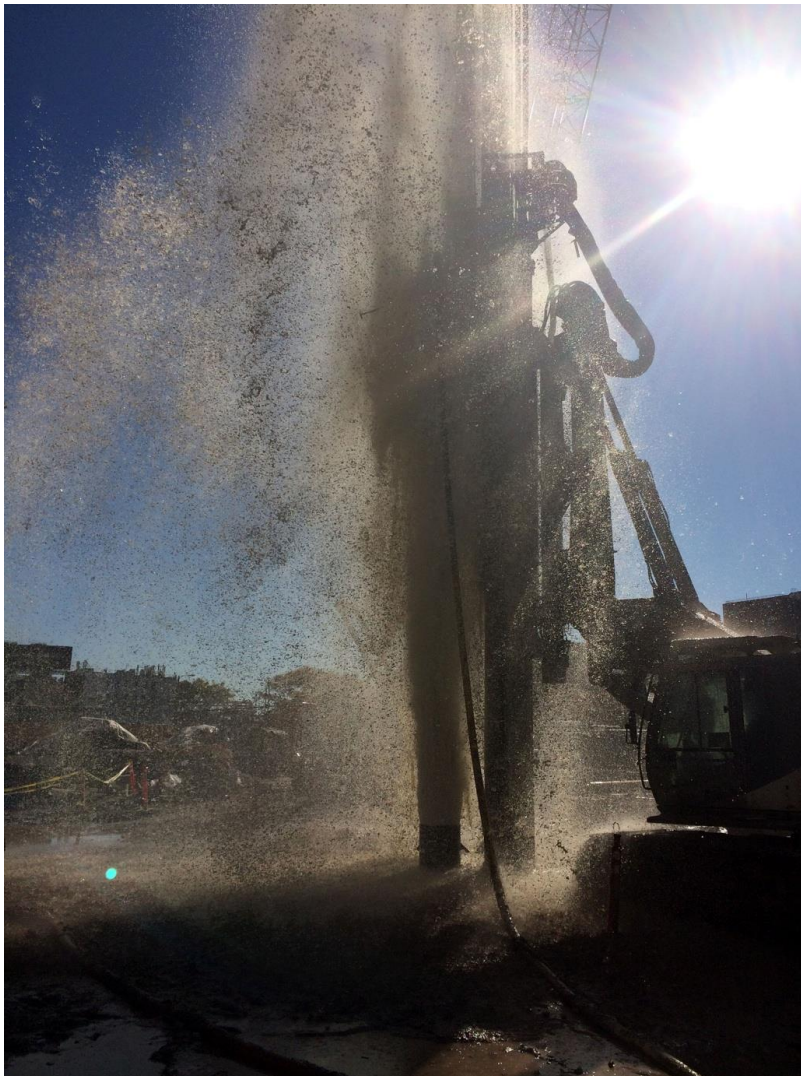
Figure 9 – View of as-built anomalous water + material flow and geysering associated with caisson drilling in November 2015 at a terrestrial caisson/pile drilling job site. (Contractor image.)
