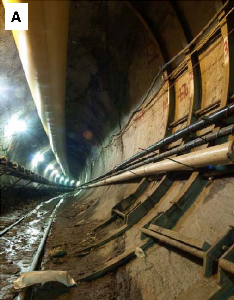
Figure 18. Photographs inside the East Side Access tunnel.
