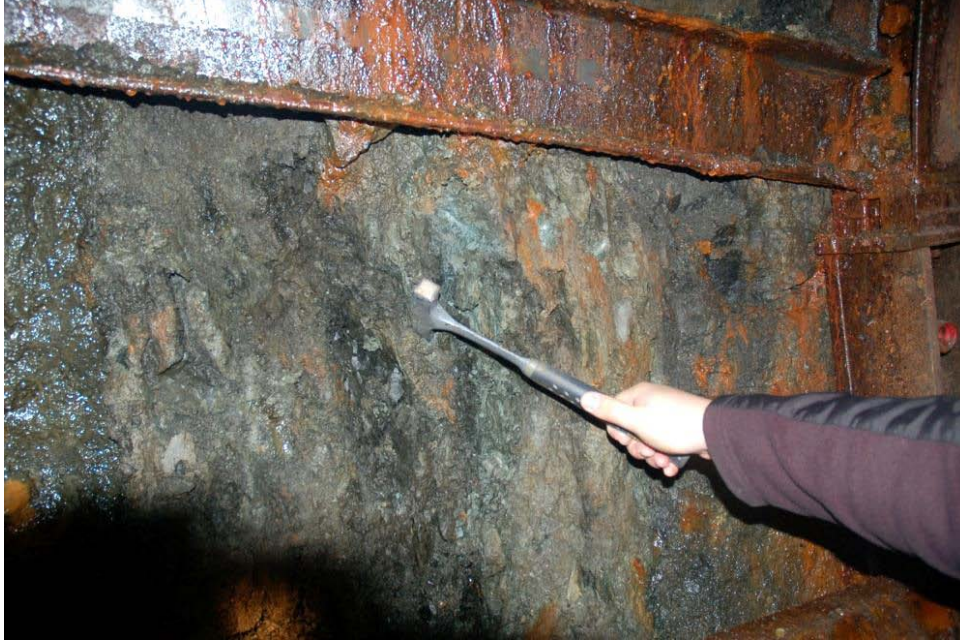
Figure 27. View of chloritic fault gouge and breccia zone associated with the Mosholu fault in the low-level treated water tunnel (Station 26+60). (Digital image by Dan Vellone.)
