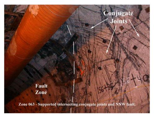
**Figure 9** – Left wall view of a N20°W fault of Group E that cuts invert at 156+35 with a 0.5 to 1.0 m thick crush breccia and adjacent area of intersecting conjugate joints (flower structure). [Image by C. Merguerian, 30 December 1998.]
