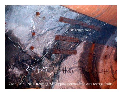
**Figure 7** – The geology of this disturbed interval (Station 214+30, left wall) is dominated by a major NNE-trending SE-dipping normal fault exposing a 3m thickness of clay-rich crush breccia. The NNE fault of Group D displaces older low-angle reverse faults (Group A) in both the footwall and hanging wall blocks of the fault. Fault splays of various orientation and offset sense are found adjacent to the NNE-fault. [Image by C. Merguerian, 18 November 1999.]
