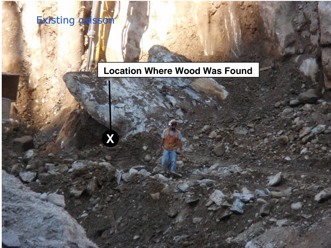
Figure 14 – Layer of silt deposited under an inclined slab of bedrock in the west depression, surrounded by till. A small tree branch was found lying on top of the till under the silt. (Digital image courtesy of D. Chen and R. Nunez.)
