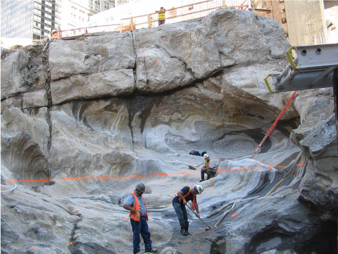
Figure 6 – Northeastern face of the western depression. The view shows an upper “cave” carved out by a whirlpool. A boring made during the geotechnical investigation cut through the upper ledge of bedrock before penetrating the till which filled the structure. A mid-level whirlpool is seen being cleared of till. Till filled potholes are visible in the upper left corner. The till was so densely compacted that sediments in the near vertical exposures remain in place. (Digital image by C. J. Moss.)
