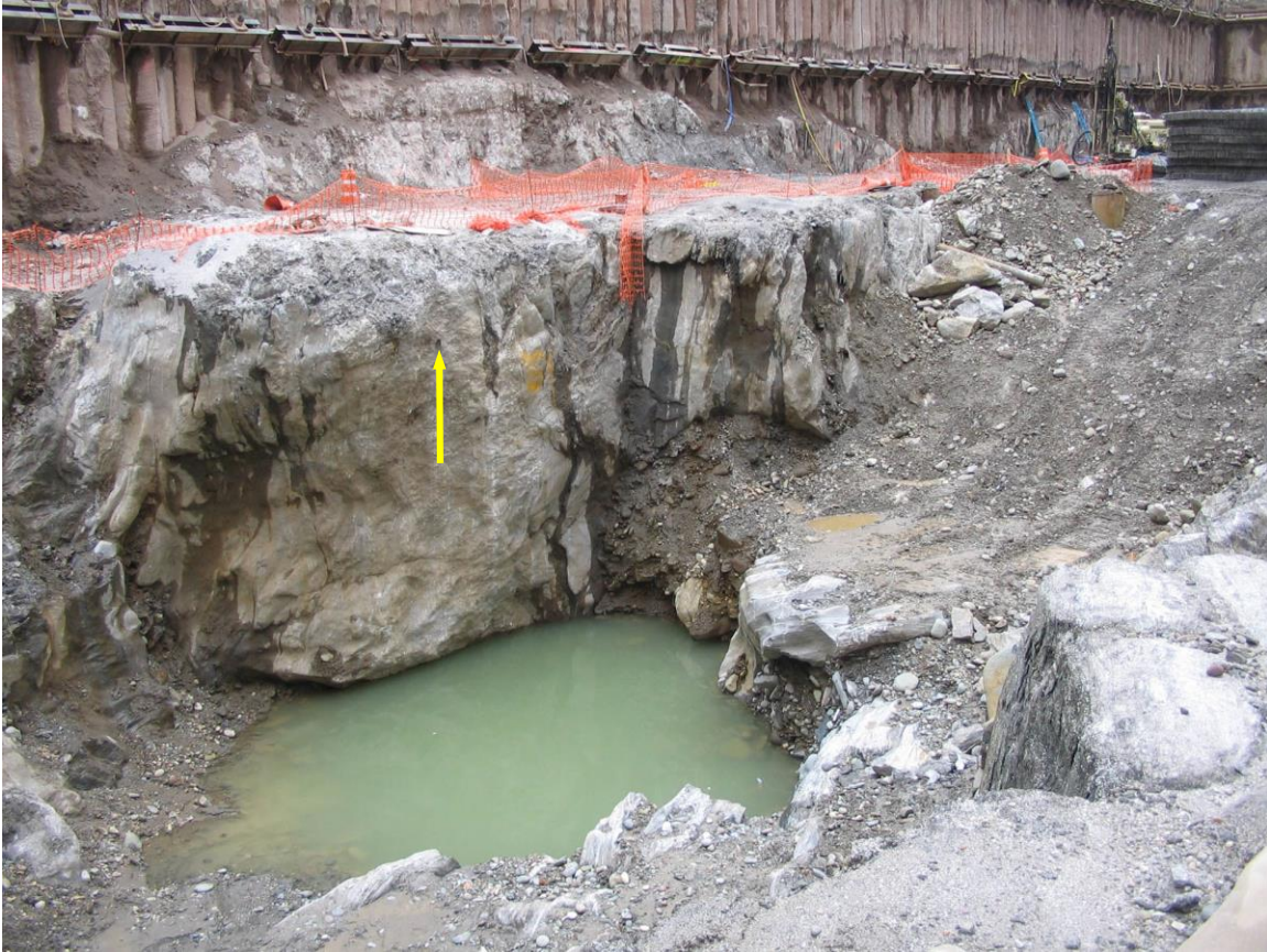
Figure 7 – Northwestern face of the west depression. At top, temporary secant wall sits above the original top of bedrock surface. Densely packed, bouldery till is seen in the center, filling a large void under the cliff face that was scoured by a plunge pool. Center right is a large, flat slab of polished, native bedrock that was originally thought to be a rock ledge until the underlying till was removed. Potholes, some still filled with till, are scattered along the sides. Green pond fills the lowest level whirlpool. Yellow arrow points to boring that cut through the upper ledge. (Digital image by C. J. Moss.)
