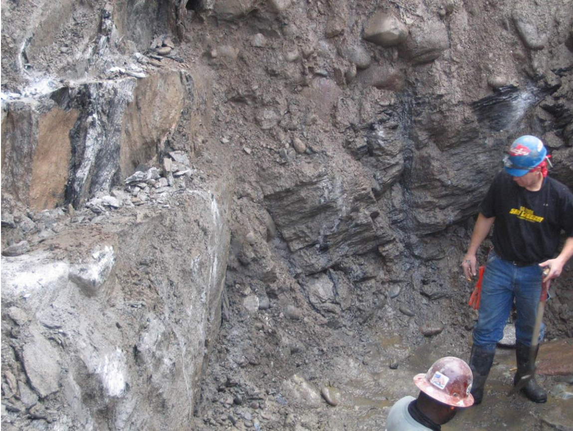
Figure 10 – Bedrock to the left shows the natural subvertical foliation. Till is to the center and right. Seen in the midst of the bouldery till is a slab of schistose bedrock that had broken loose and tipped to the side as it was incorporated into the mix. (Digital image by C. J. Moss.)
