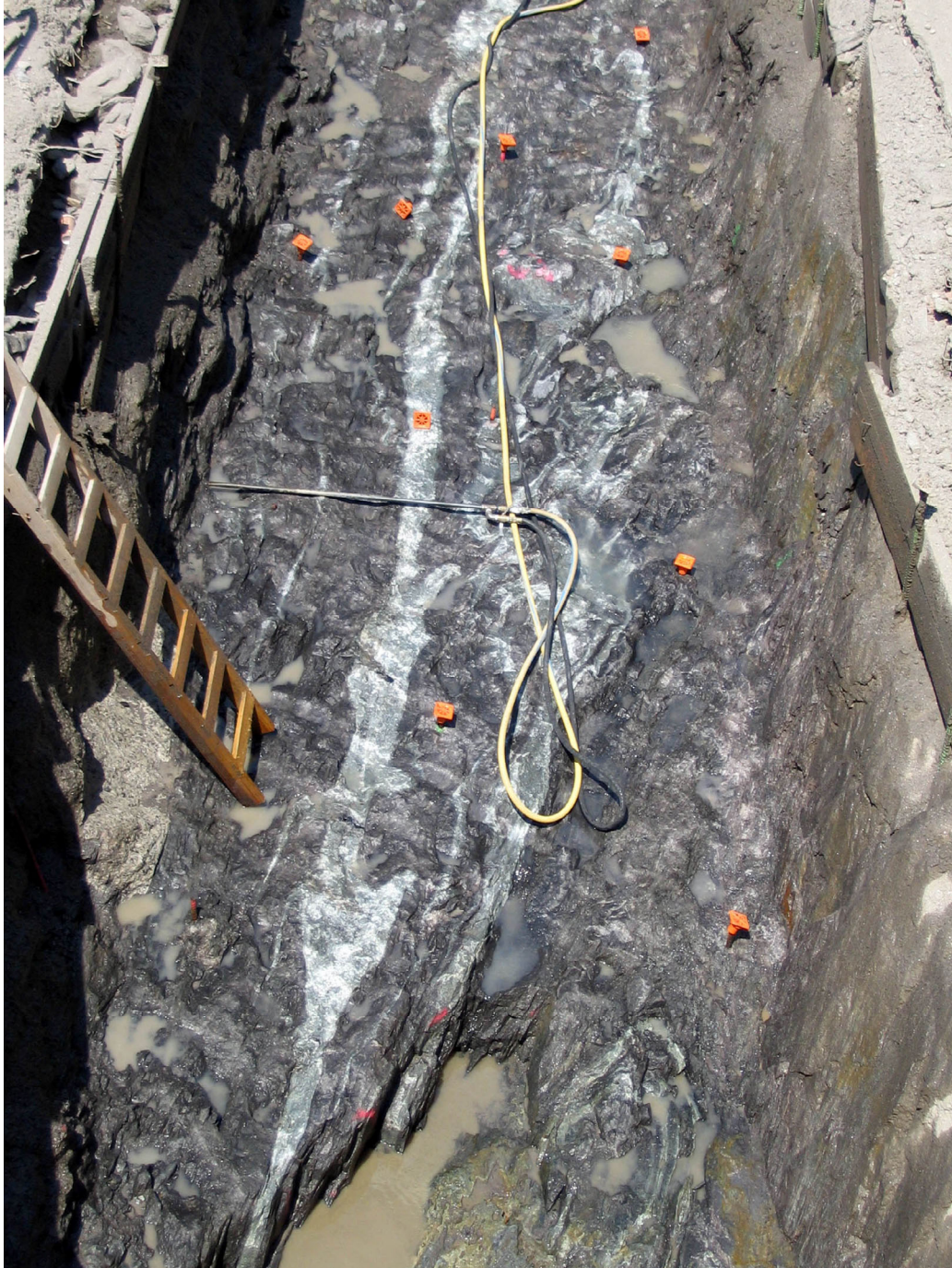
Figure 3 – Vertical asymmetric fold of Walloomsac calc-silicate and interlayered schist found in an excavation along the eastern edge of the west bathtub. (Digital image by C. J. Moss.)
