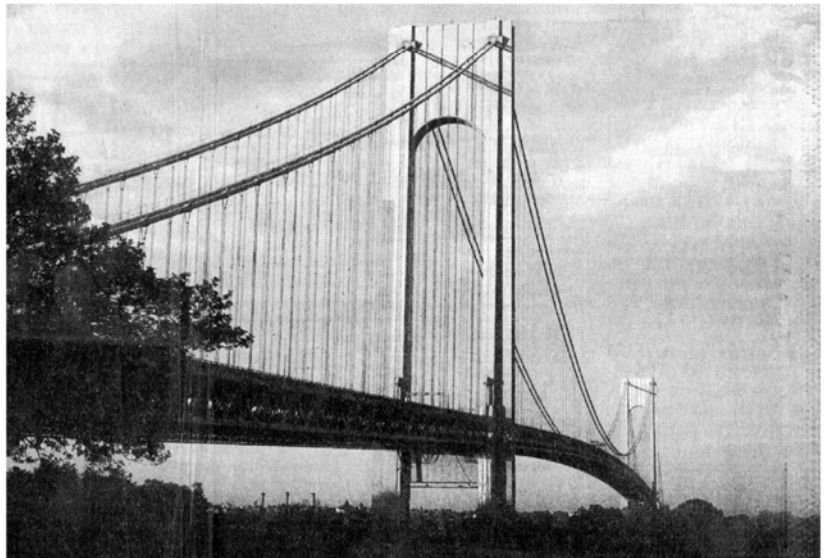
Construction work caused a traffic slowdown on the Fingerboard Road ramp to the Verrazano-Narrows Bridge recently due to the installation of earthquake-resistant bearings, part of a statewide bridge rehabilitation program.
