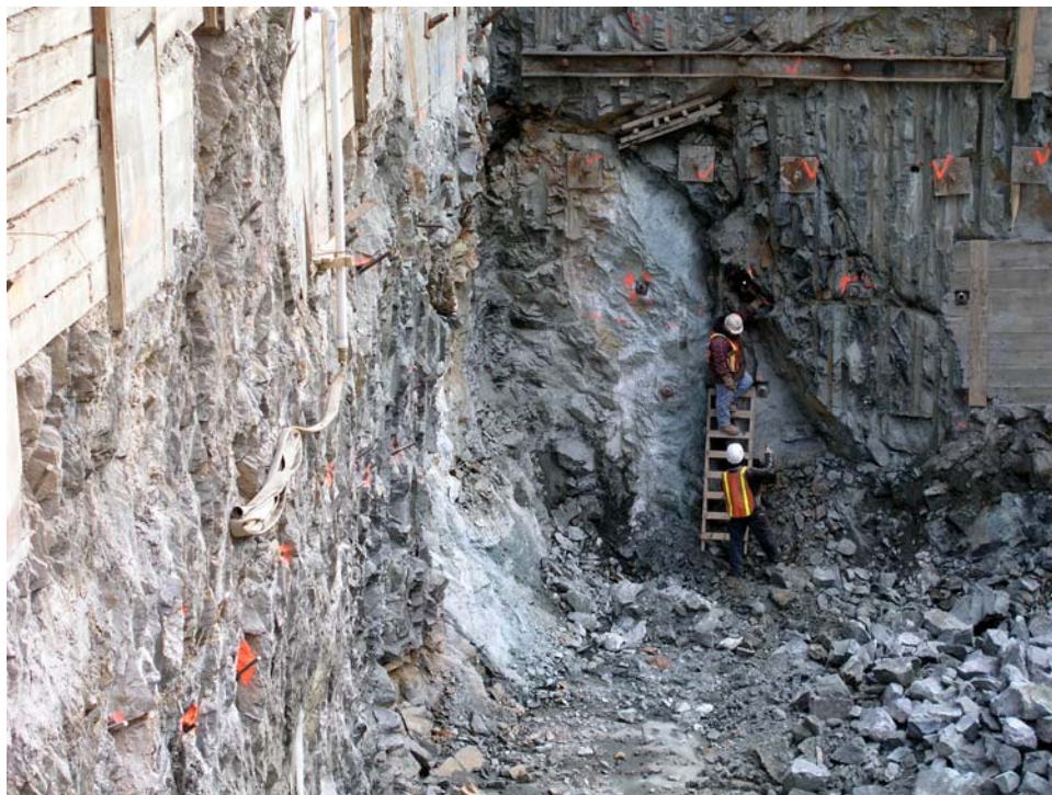
Figure 2 – View toward the ENE of top portion of zoned serpentinite found SW of the corner of 43 rd Street and Sixth Avenue in Manhattan. The body exhibits a dark-colored massive serpentinite core, light green talc schist and outer biotite schist zones and surrounding massive amphibolite. Digital image taken 21 December 2004.
